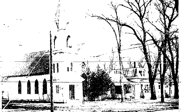
The old St. Mary's Catholic Church, as we know it, will soon be a thing of the past. Dormer windows will appear in the roof and new windows and siding will help transform the still serviceable building into an apartment house.
